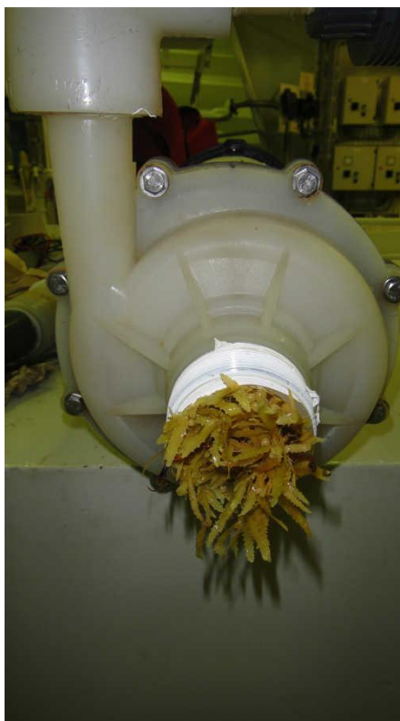
Figure 1: Explorer of the Seas environmental monitoring system seawater pump clogged with Sargassum weed.
