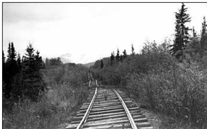
Figure 1: Permafrost damage to Copper River and Northwestern Railway in Alaska. Source: http://earthdata.nasa.gov/sites/default/files/styles/large/public/2005_permafrost_copper.jpg
