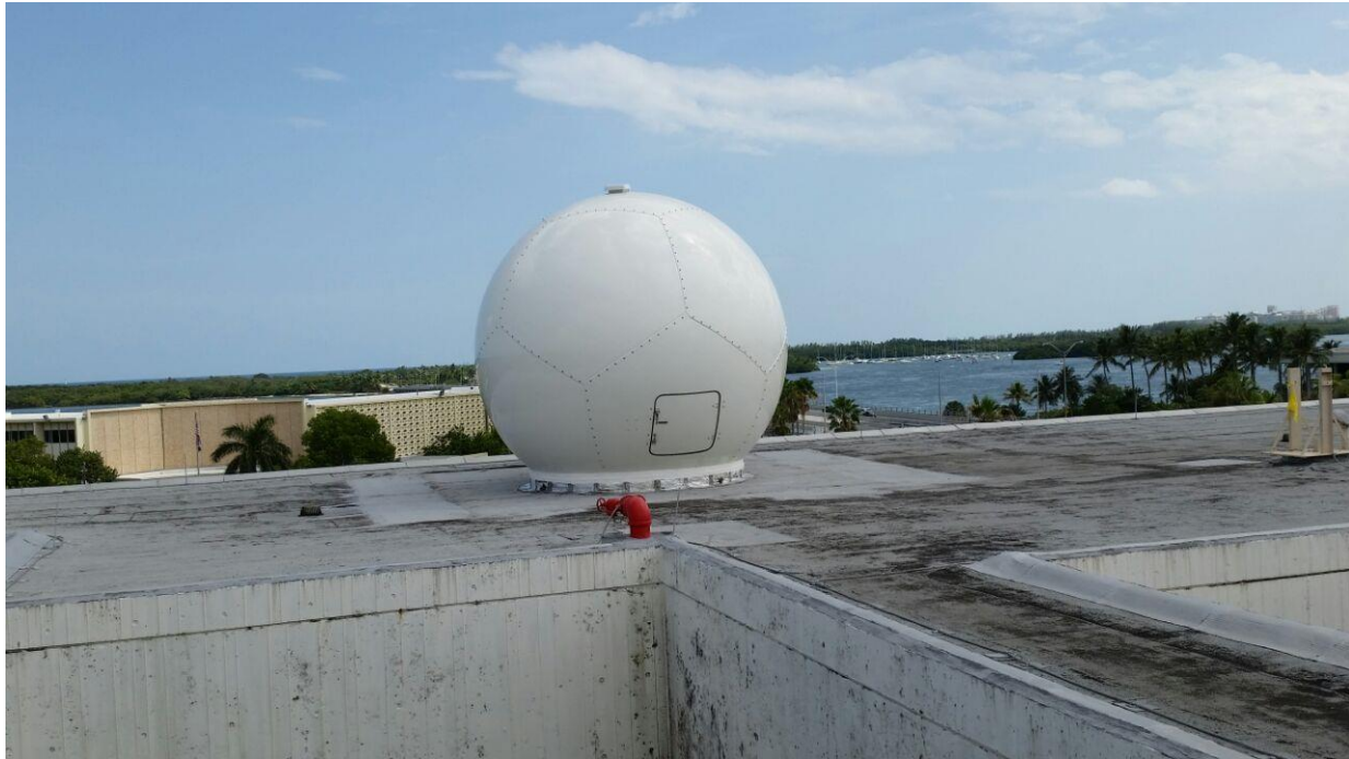
Figure 1: New X-Band antenna on AOML's roof. It is protected from the environment by a radome, certified to 155 mph. The new system is capable to receive telemetry from the Suomi-NPP satellite and the future JPSS satellite missions.
